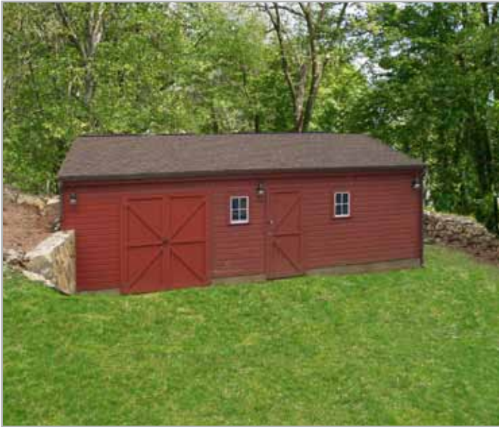
The Barn with electricity, water, cable and phone.
