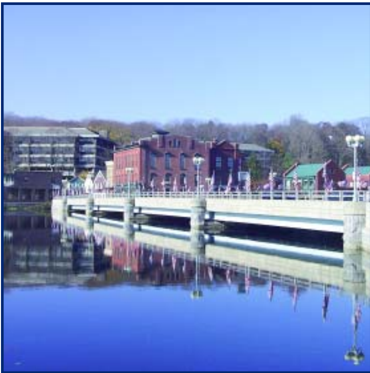
Saugatuck River Bridge to Main Street.
